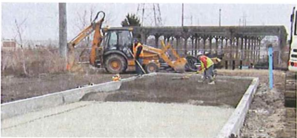
Backfill installation on top of deck.
