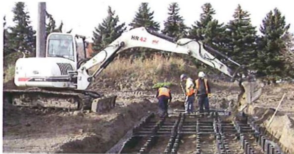
Soil cell trench filled with soil
