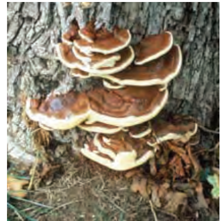
Figure 3.9. Fungal fruiting bodies indicate advanced decay.
